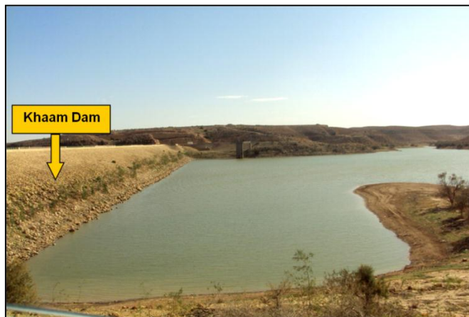
Figure 6. Showing the Formation of Ka'am Lake in front of Ka'am Dam.
