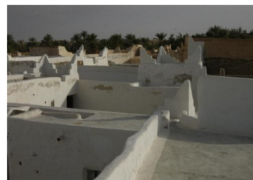
Picture 4. A view from the roofs shows the windcatchers on the kitchens' roofs
