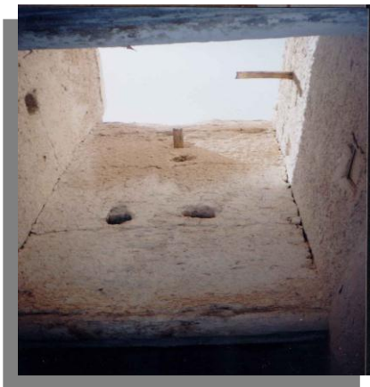
Picture 5. An interior view of a lighting shaft from the street
